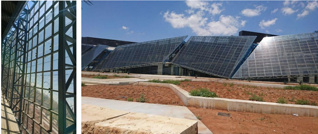
Building Integrated Photovoltaic System (BIPV)
