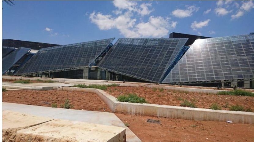
Building Integrated Photovoltaic System (BIPV)
